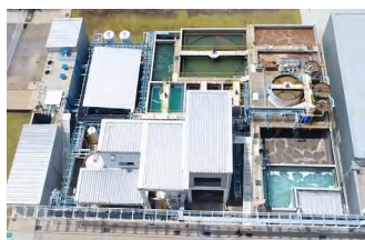
Wastewater recycling plant (MMTh)
