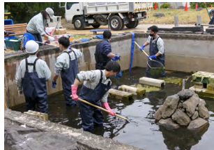
Employees engaged in pond draining and cleaning
