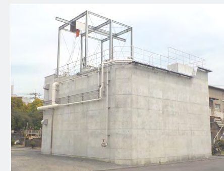
Sewage and domestic waste water processing facility (Mizushima Plant)
